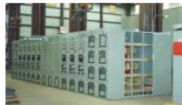
Low Voltage Generator Control with 12,000A Main Bus Generator Control Switchgear for Parallel of 10 – 480VAC Generators Oxy Oil and Gas Ecuador
